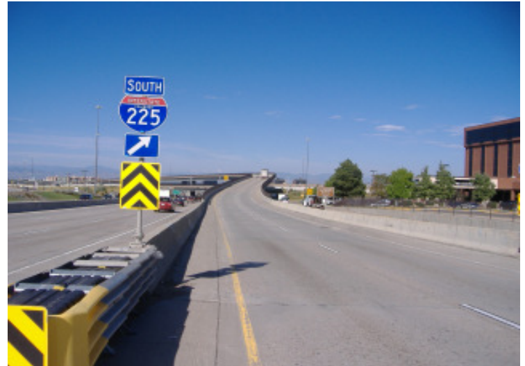
The ramp from northbound Parker Road to southbound I-225 will have added traction for the winter (Project #20).
