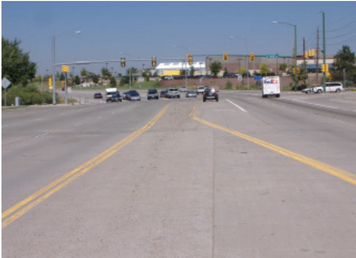
A third through lane will be added on northbound Parker Road at Orchard Road (Project #19)
