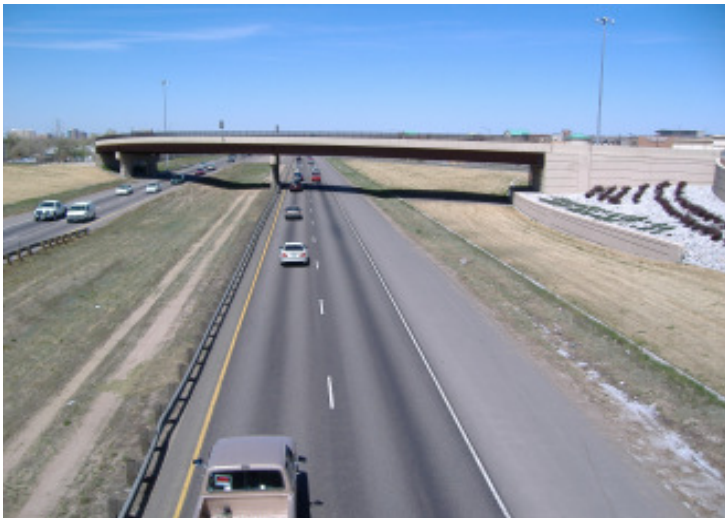
A third through lane in each direction of I-255 between Mississippi Avenue and 2nd Avenue will improve traffic flow (Project #23).
